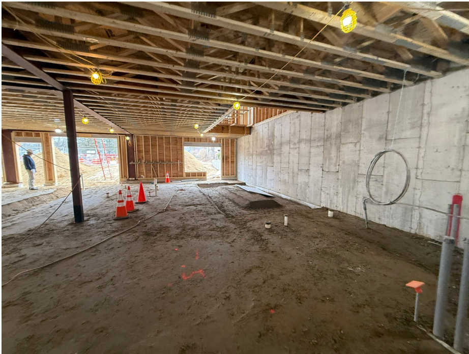
Interior framing taking shape inside the new building — foundation walls in place, beams set, and rough openings ready for windows.
