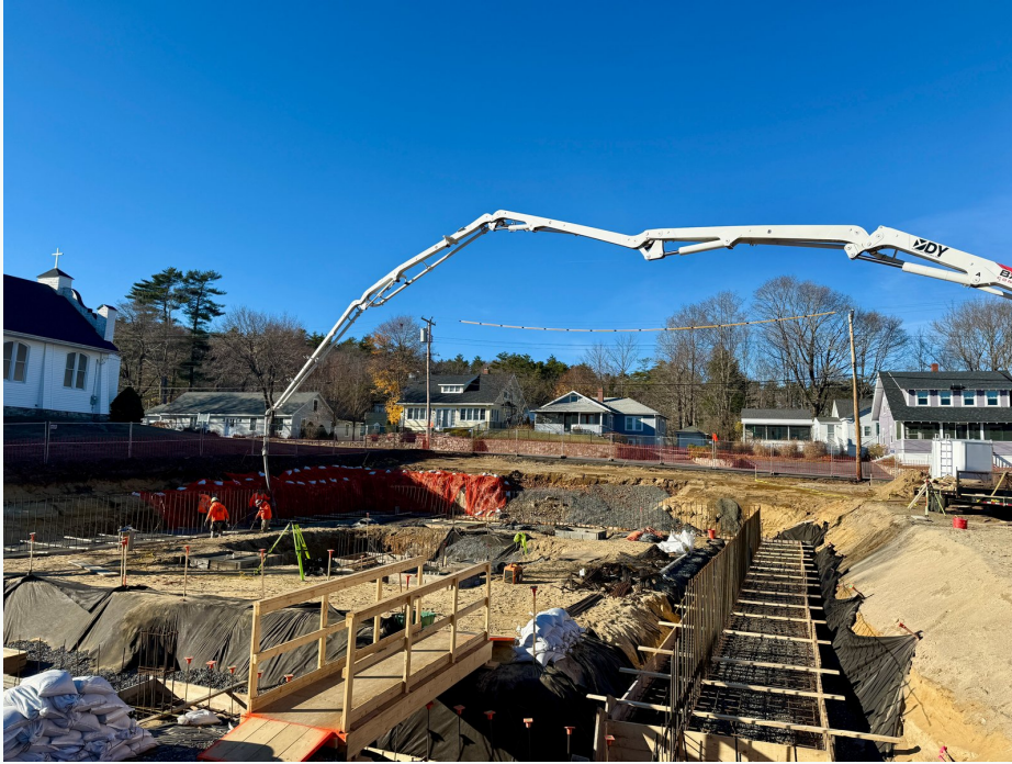
Concrete pump at work on the Municipal Campus foundation pour — the largest single capital project of the year.
