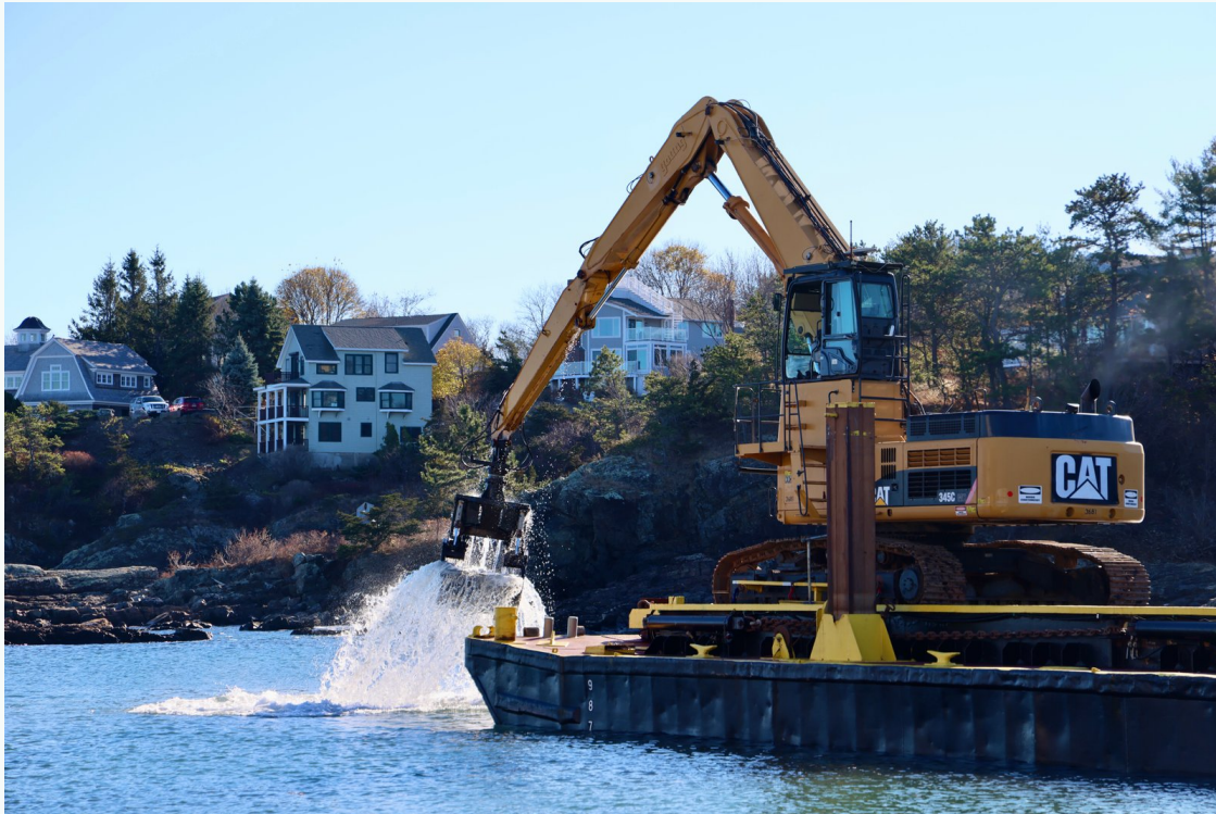
Perkins Cove Dredge in progress — work was completed in March 2025, restoring depth and access for the working waterfront.
