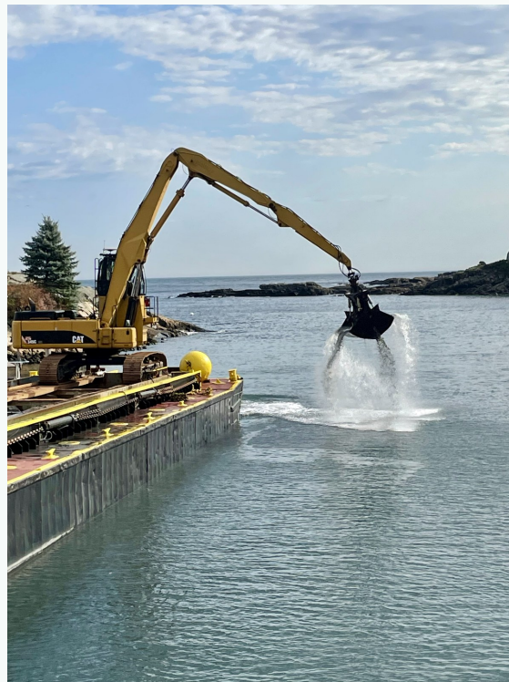
The dredge bucket at work in Perkins Cove, November 2024.
