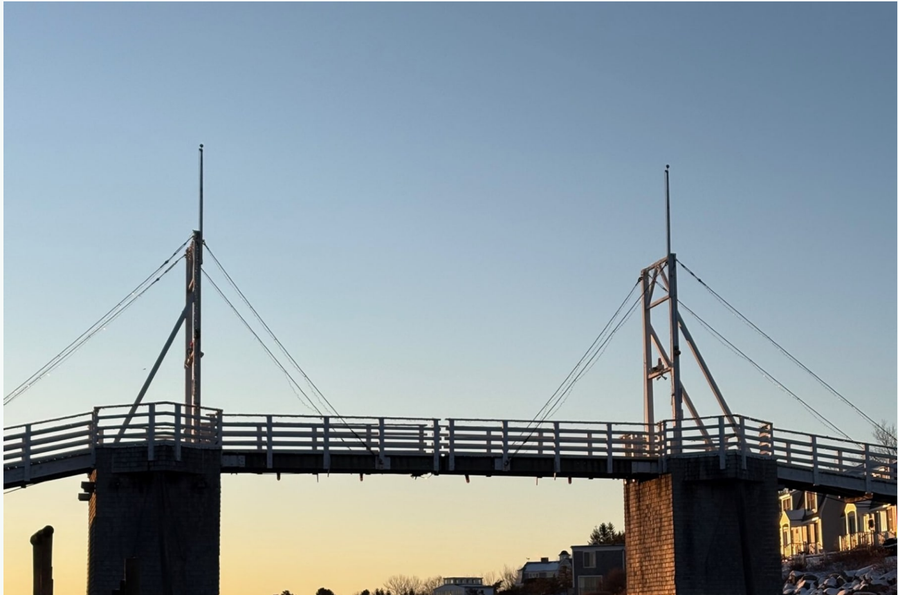
Perkins Cove footbridge at winter sunset, 2024–2025
